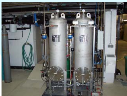
Figure: Filter systems designed for a flow rate of 1 l/s and 50 l/s.
